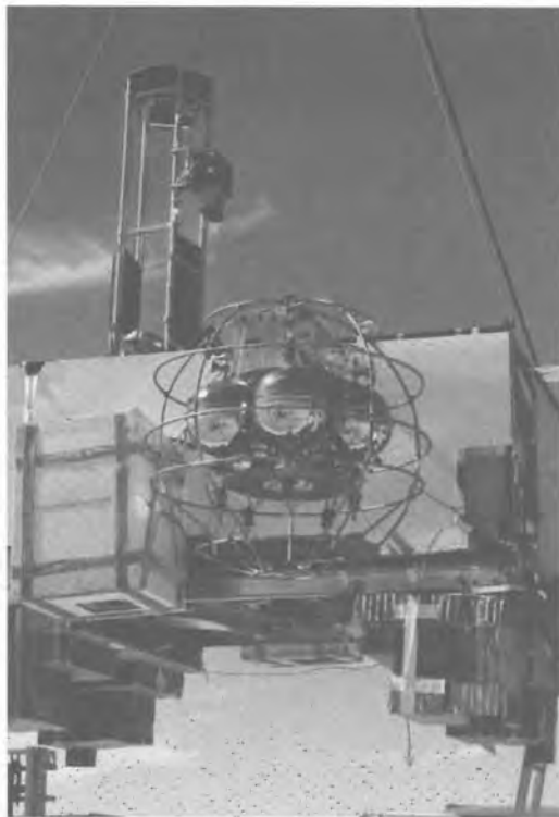
Fig. 68. (Right) Payload launched by an Air Force high altitude balloon from Holloman AFB, N. M. on March 20, 1965. This payload was a scientific experiment for The John Hopkins University Astrophysics Laboratory. (U.S. Air Force photo)
