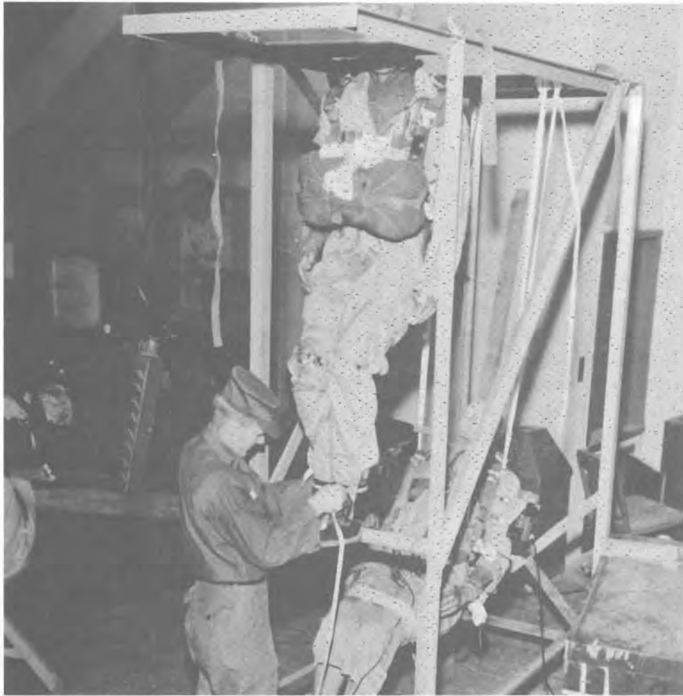
Fig. 75. "It's uniform was torn in a couple spots...their uniforms were in pretty sad shape"—witnesses description of secondhand flightsuits that were used repeatedly on tests; tears and other damage were common. In this photo, 1st Lt. Raymond A. Madson "rigs" a dummy to its suspension rack for project HIGH DIVE at Holloman AFB, N.M. (U.S. Air Force photo)
