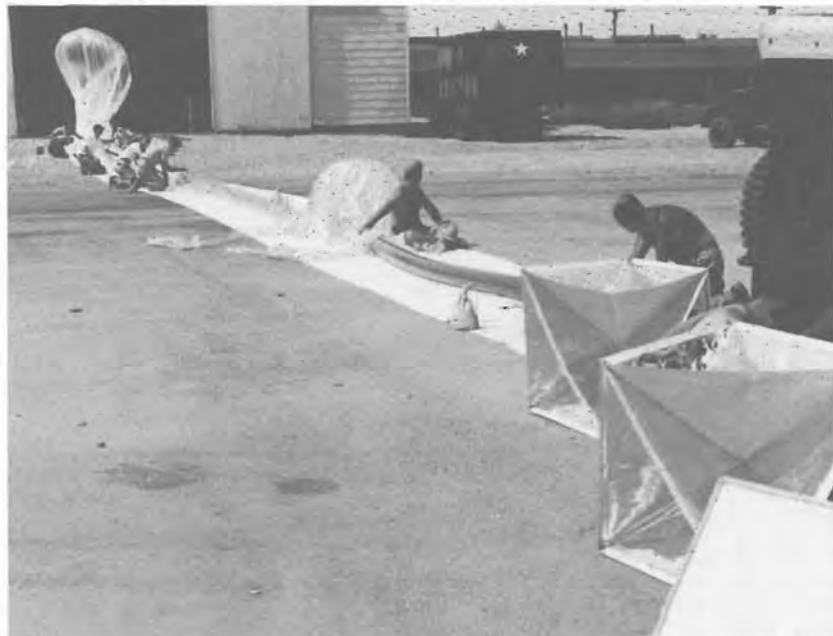
Fig. 5 & 6. (Below, left and right) Constructed of aluminized paper glued and taped to a balsa wood frame, several ML-307B/AP radar targets were used on the MOGUL balloon train to make it visible to radar. (U.S. Air Force photos)
